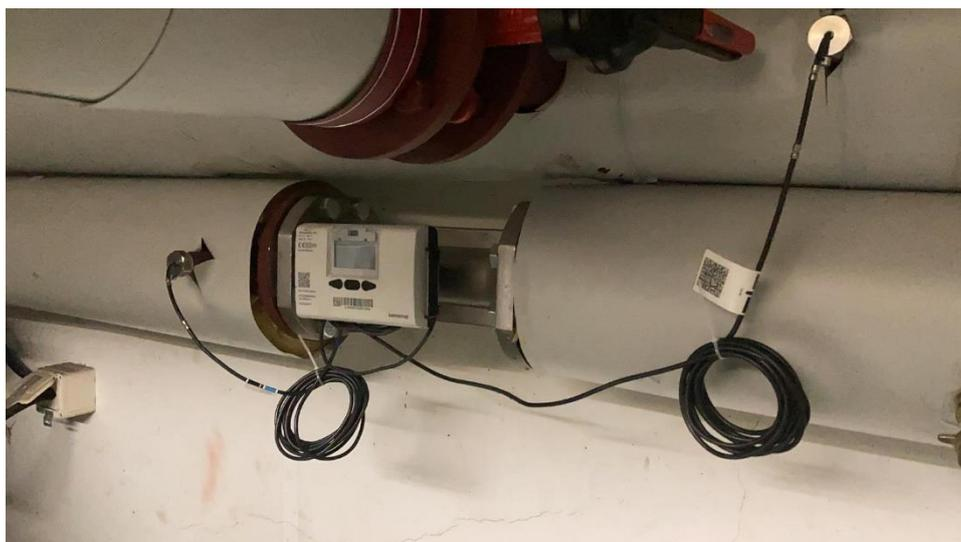
**Figure 12: B1.3: Installed heat counter**
