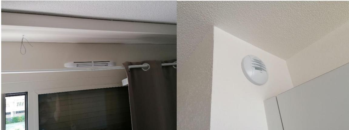
**Figure 4: Humidity-sensitive inlet and exhaust valves installed in B1.3**
