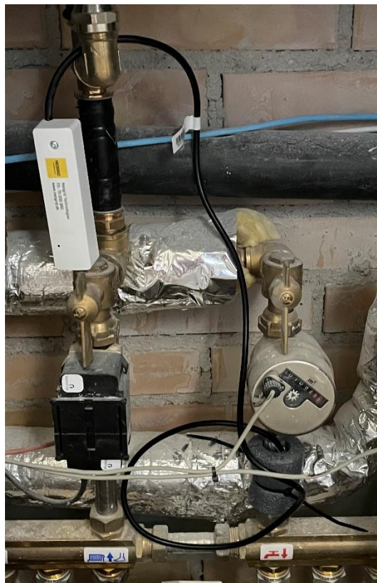
Figure 31: Simple indoor climate sensor (temperature & humidity) with external probes for pipes
