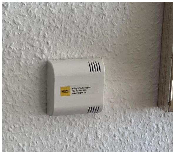
Figure 29: Indoor climate sensor with CO 2 measurement
