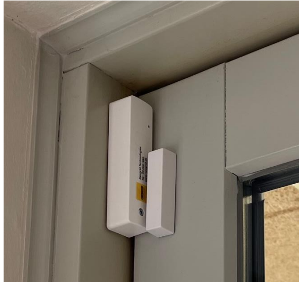
Figure 30: Contact sensor measuring door/window opening
