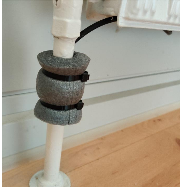
Figure 32: Contact sensor mounted on a radiator pipe in the apartment
